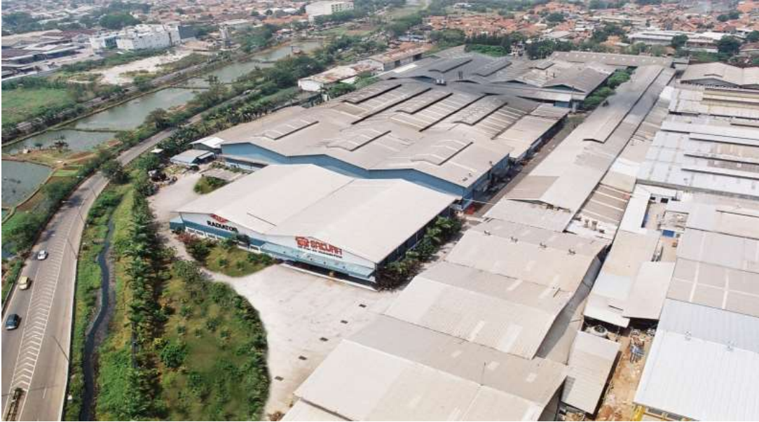
Kapuk Plant (Radiator Facilities)
